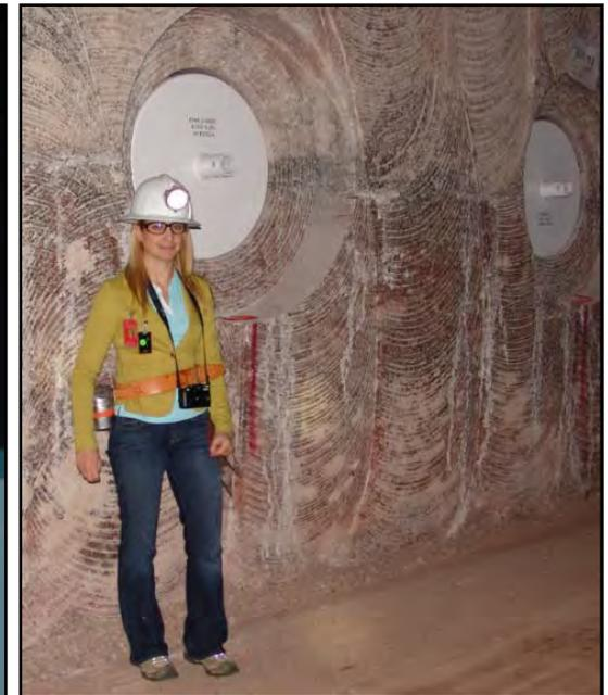
Photo 2: Room 6, plugged horizontal borehole for Remote Handled Waste
