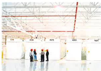
Used Fuel Dry Storage at OPG Western Waste Management Facility (Ontario)
